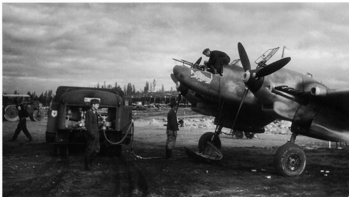
As the enlarged oil cooler and sand filter on the supercharger intake show, this is a Bf 110 E modified for tropical service. This is, in fact, the only tropical early series Bf 110 known to have served with JG 5, but unfortunately the code is not known. The sub-type can be determined by the air channel just discernible on the dorsal part of the MG cover lying on the ground beneath the aircraft. This was part of the new heating system introduced in the Bf 110 E series. The camouflage comprises the normal greys (BA).
