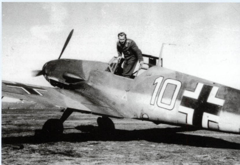
A very revealing photograph of 'Yellow 10' of Lt. Hans Döbrich. As can be seen, there are at least three different upper surface colours; RLM 79 around the cockpit (note canopy frames are in original paint), a slightly darker colour (RLM 75) behind the number and a darker colour above and in front of the fuselage cross (thinned RLM 70 or RLM 71?) and RLM 70 on the nose and over the top part of the white tail band. The lower part of the tail band have definitely been retained and there are traces of a lighter colour around the numeral where it overlaps the blue under surface colour, this is almost certainly RLM 76. The fact that the frame numbers and black outline of the foot step are retained is significant, this proves that the bottom and part of the side surfaces are still finished in the factor-applied colour of RLM 78 (Coll. Döbrich).
