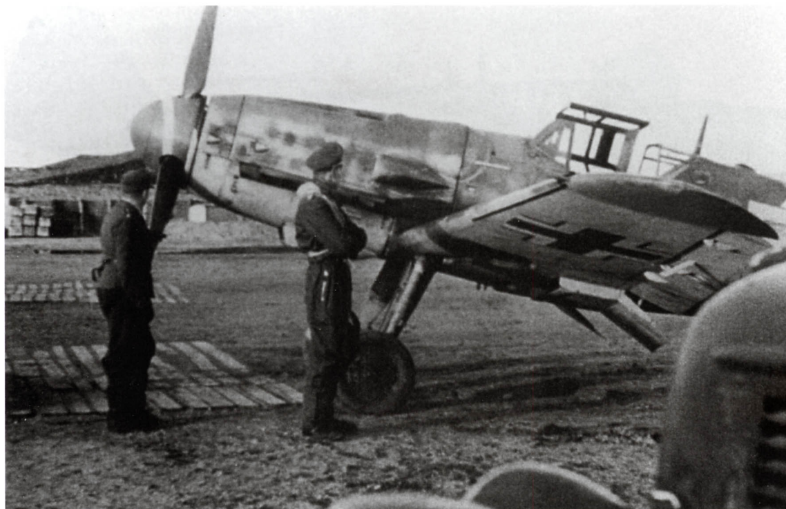
Allegedly showing Oblt. Kurt Schulze's 'Yellow 5' from 9./JG 5, this mid-production G-6 (note short antenna mast and DF loop base) was probably typical of III./JG 5 G-6s in the summer of 1944. The camouflage is in the regular grey with fairly heavy mottling on the fuselage sides. The spinner is probably black-green with a white spiral. Note the yellow outer wing panels (Coll. Horst Kube).
